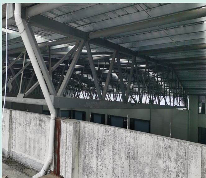
Photo of the newly installed atrium roof
