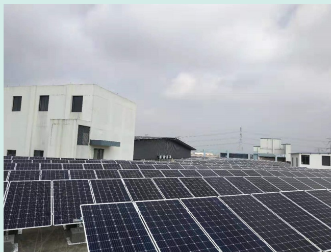
Solar panel installation at Fu Heng Warehouse, Hangzhou City
