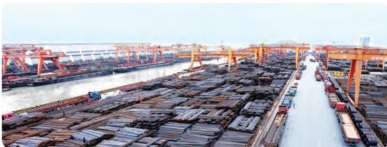
Stockyard for steel products at Chongxian Port Investment
